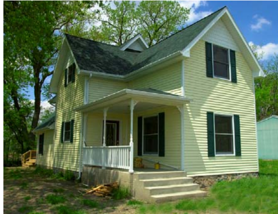
Turn of century home along Tippecanoe River after renovation
