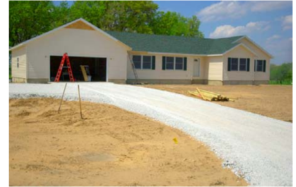
Holmes' home under construction in Phase I
